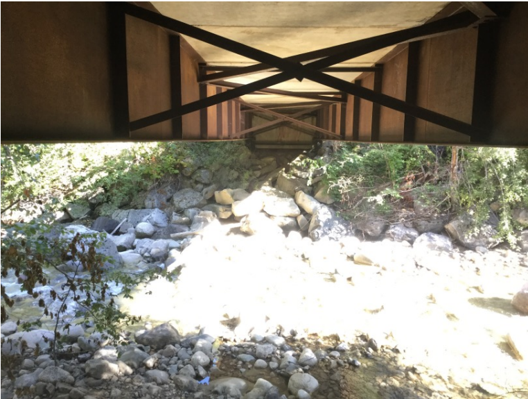
Right Bank Abutment when facing downstream
