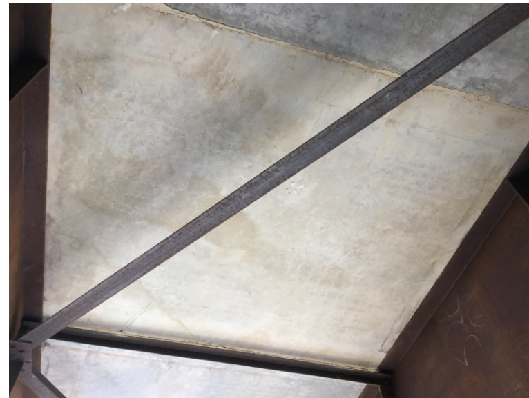
No cracking visible under panel
