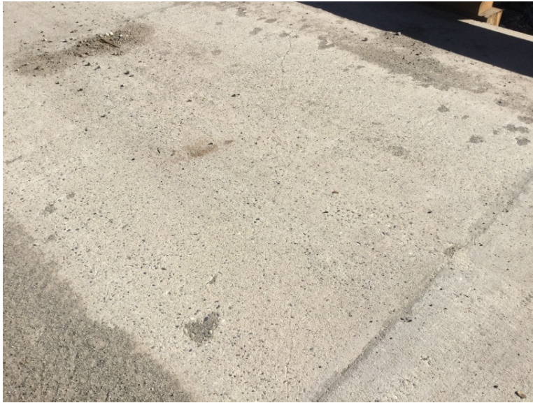
Crack in deck panel
