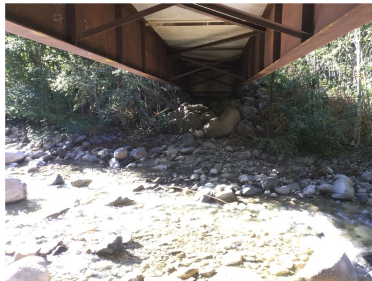
Left Bank Abutment when facing downstream
