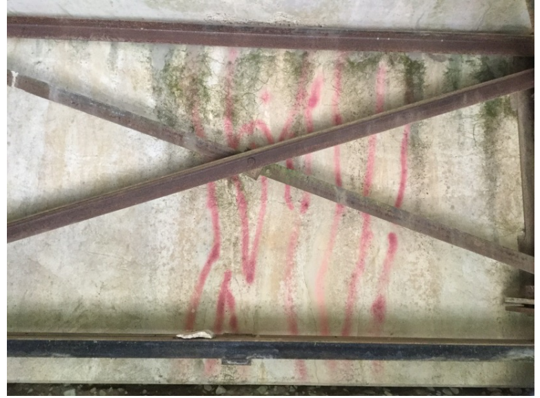
Ballast wall at right bank
